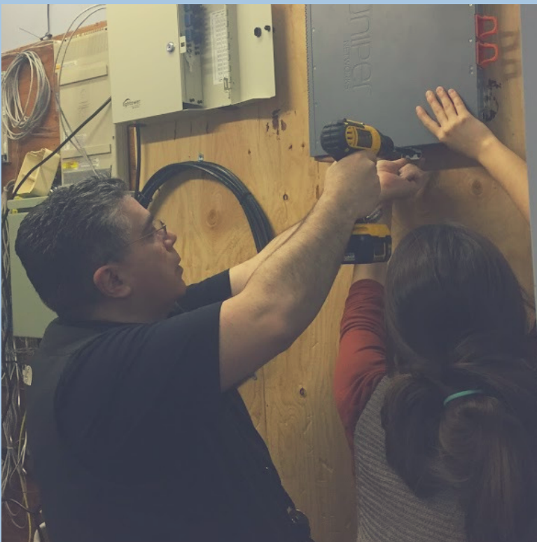
CEN representatives installing new equipment.
